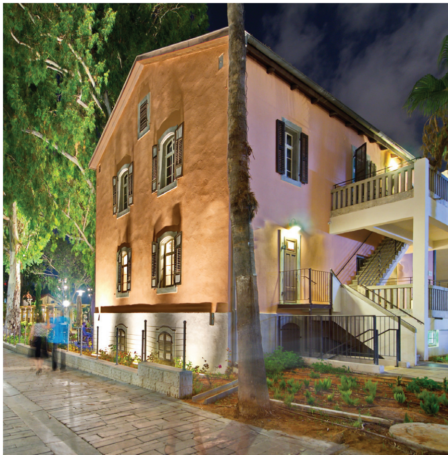
Restored House in Saron, Tel Aviv
