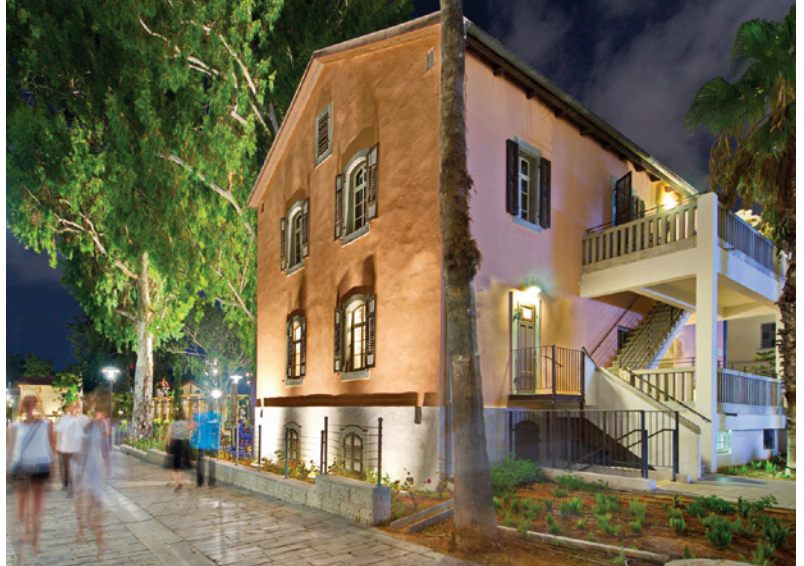
Restored house in Saronia, Tel Aviv
